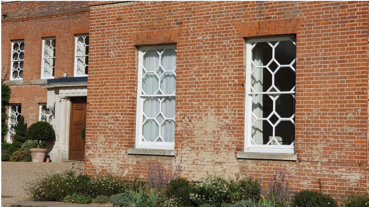
Figure 1. Windows at Braxted Park, Essex.
