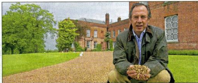
● CUTTING COSTS – Duncan Clark, owner and manager of Braxted Park, with wood chips used to feed the new boiler.
